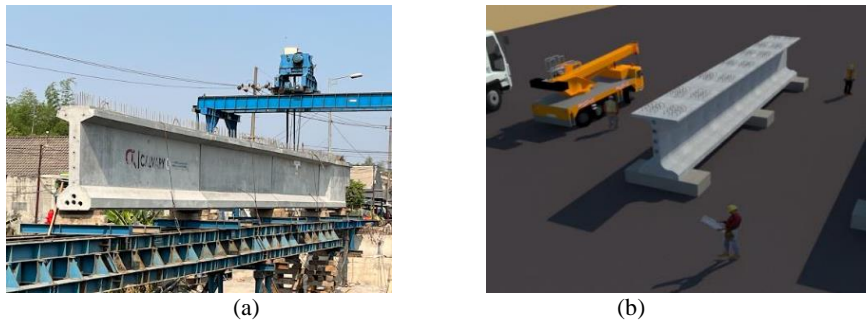
Gambar 4. (a) Levelling girder metode perancah (b) Levelling girder metode launcher
