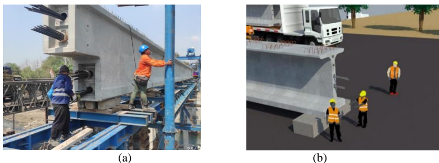
Gambar 5. (a) Install PC strand metode perancah (b) Install PC strand metode launcher
