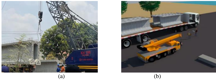
Gambar 3. (a) Supply girder metode perancah (b) Supply girder metode launcher
