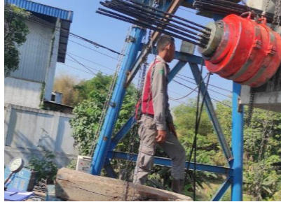
Gambar 6. Stressing girder metode perancah
