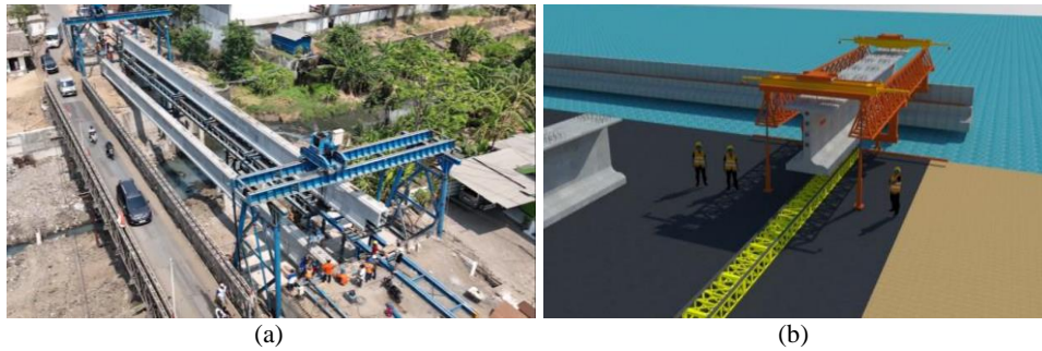
Gambar 8. (a) Erection girder metode perancah (b) Erection girder metode launcher
