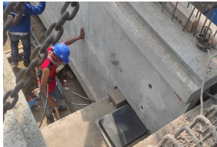
Gambar 7. Grouting dan patching girder
